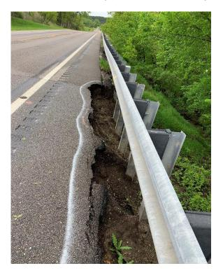
Figure 6. Washout Area at the Guardrail
