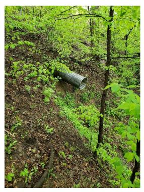
Figure 7. Erosion at the Culvert End
